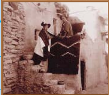
Pueblos, built of sun-dried brick, or adobe, were characteristic dwellings of the Southwest.
