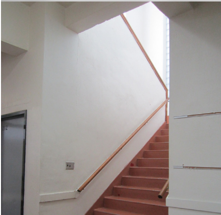
Noncompliant handrail in exit stairwell
