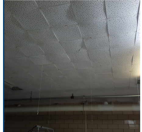
Stained, punctured, cracking and uneven ceiling tiles
