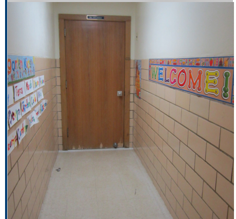
Limited maneuvering clearance on the pull side on the south side classroom doors
