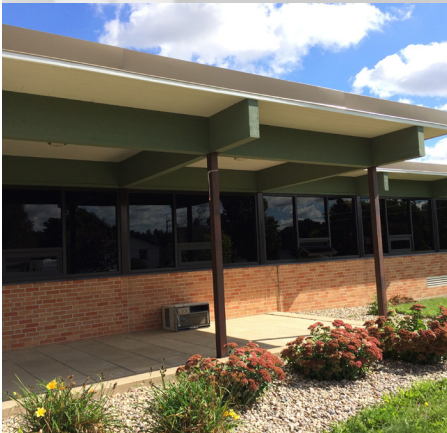
Exposed wood roof framing system
