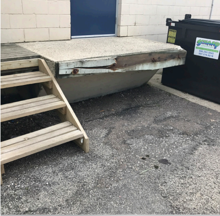
Exposed and rusted rotting wood on bolts and dowel bar
