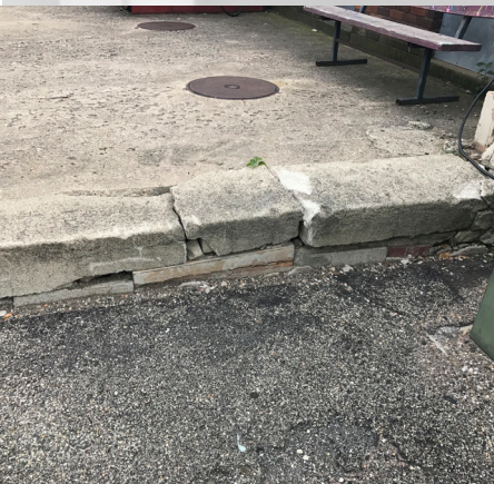
Cracking, pitting and two-foot drop along the western side of the pavement
