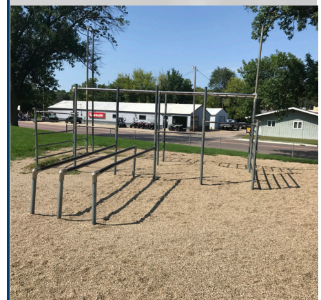
Rusting, discoloring, scraping, and missing pieces on metal playground
