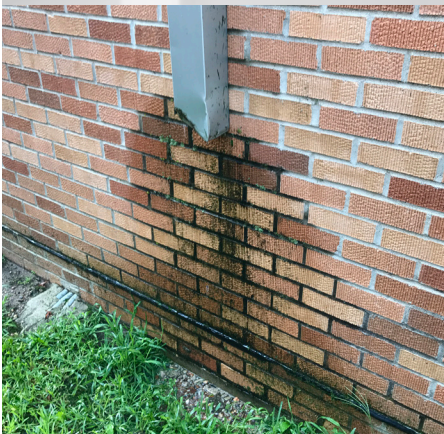
Splash block missing on roof drainage
