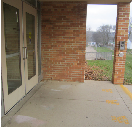
Elevation difference in stoops and sidewalks
