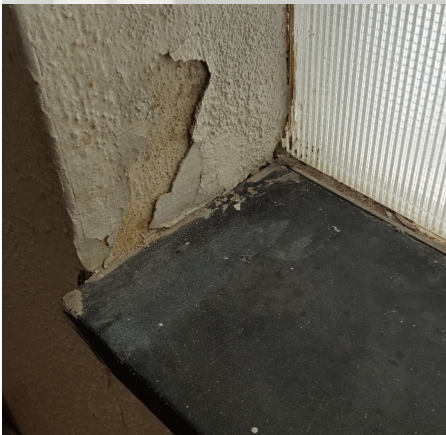
Damaged plaster wall
