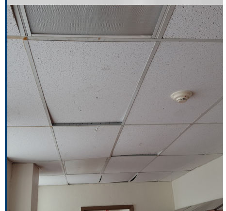
Stained and warped ceiling tiles
