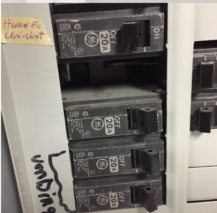
Branch panel missing blank space covers
