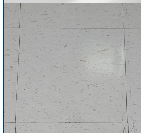
Vinyl composition tile with localized cracking and evidence of wear
