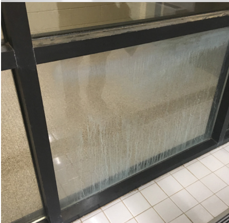
Broken seal in pool area window
