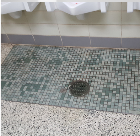
Staining on tiles under urinals.
