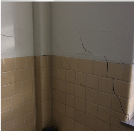
Cracks in wall of upper level
