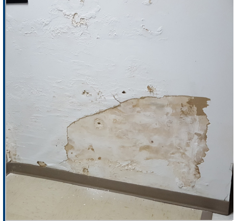
Localized damage in plaster wall
