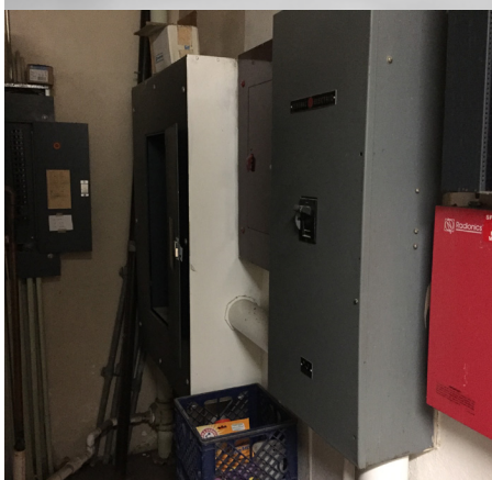
Main switchboard without proper working clearance
