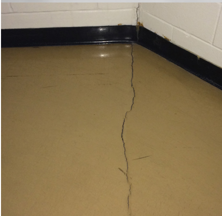
Cracked floor by track around Gym
