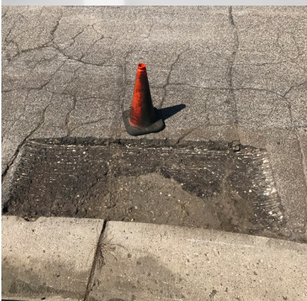
Patching of pavement being performed in circulation access of parking lot B
