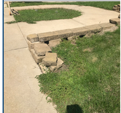
Loose bricks on northern retaining wall
