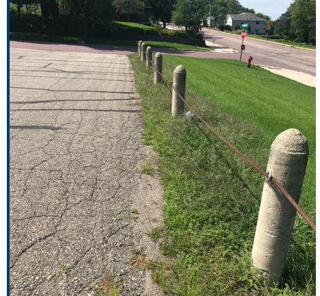
Minor sediment buildup along the north pavement/grass edge
