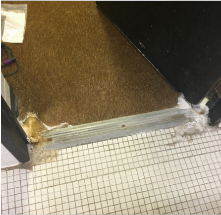
Chemically damaged carpet and tile
