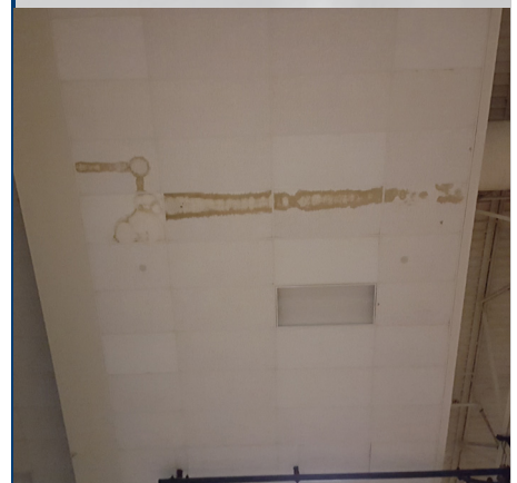
Ceiling tile with moisture staining
