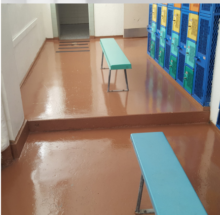
Unmarked elevation differences on concrete locker room floors
