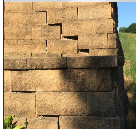
Damaged retaining wall
