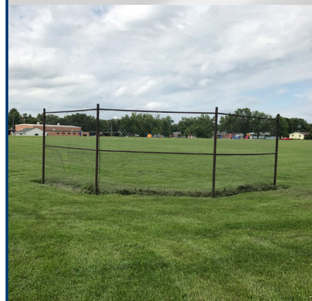
Rust and hole in chain-link baseball backstop fence
