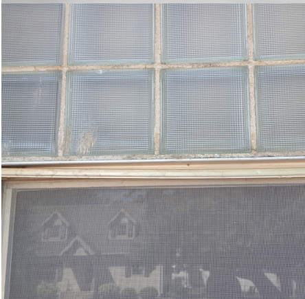
Bent frames on window system
