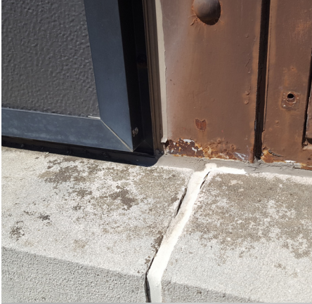
Rust and joint failure on metal framed window systems
