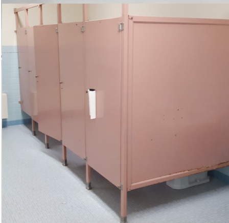
Chipped and rusting at seams in metal partitions
