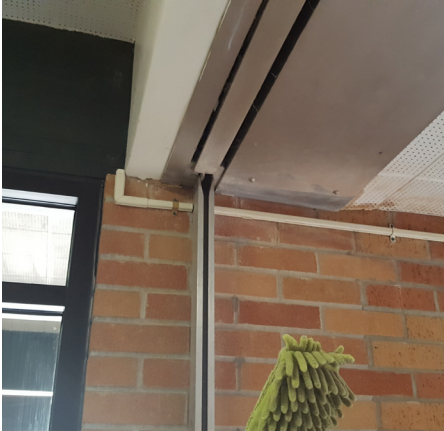
Recessed ceiling security grille
