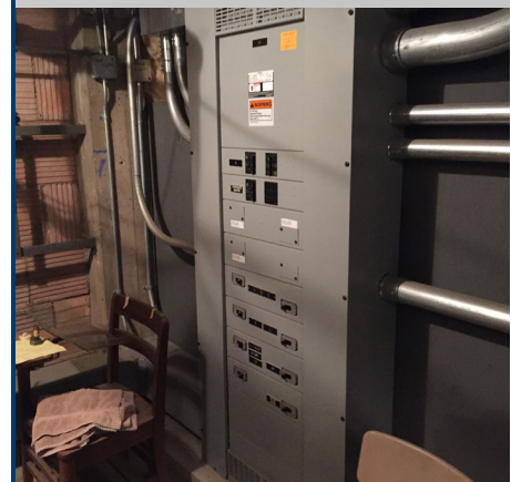
Distribution switchboard
