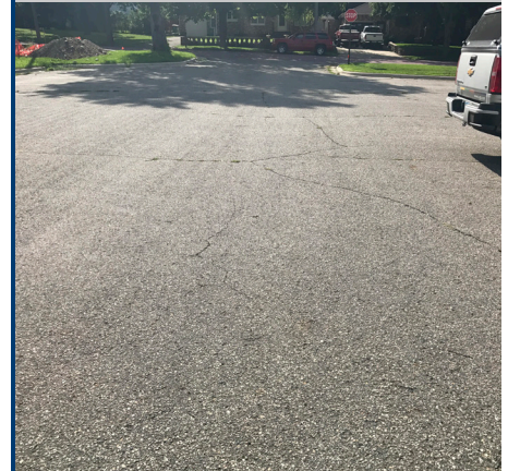
Minor longitudinal / transverse cracking with growing vegetation in pavement in southern parking lot
