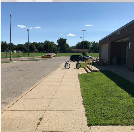
Minor cracking and vegetation growing through the panel joints of sidewalk
