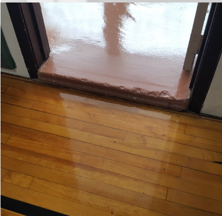
Noncompliant riser in exit stairs
