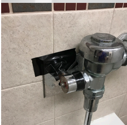
Broken flush valve on urinal
