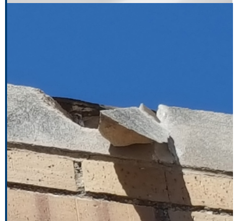
Concrete cap breakage
