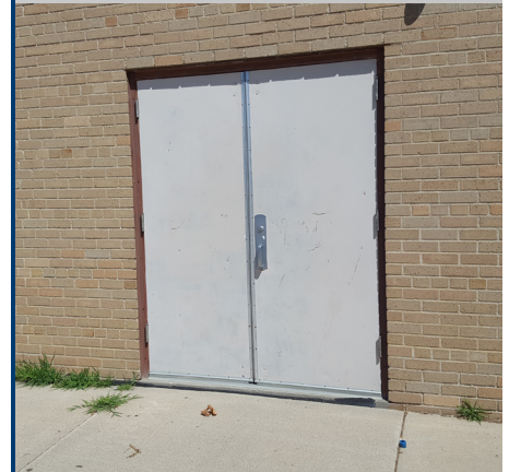
Elevation differences in stoops and sidewalks in exterior doors
