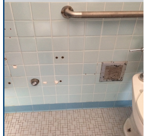
Joint stain, damage where items previously attached in glazed concrete block wall
