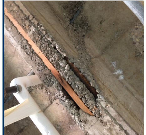
Exposed Rebar in Joint
