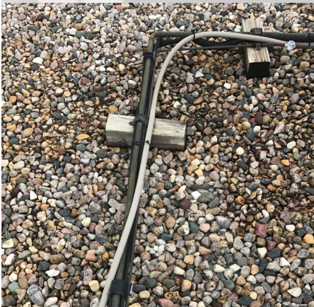
Refrigerant piping insulation is missing
