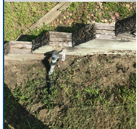
Exposed and damaged utility line
