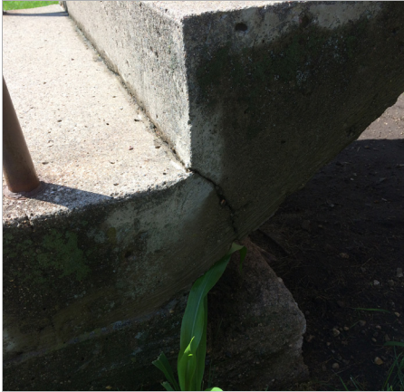
Concrete stair cracks
