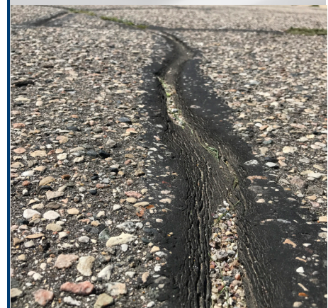
Previous joints losing seal and loss of aggregate in parking lot D
