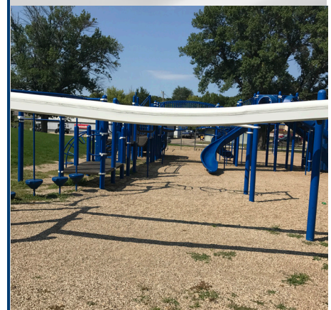
Bowing in center of track equipment
