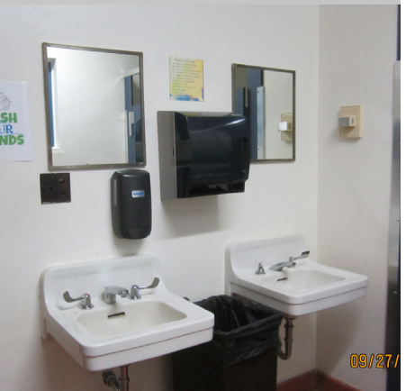
Noncompliant mounting heights in restroom
