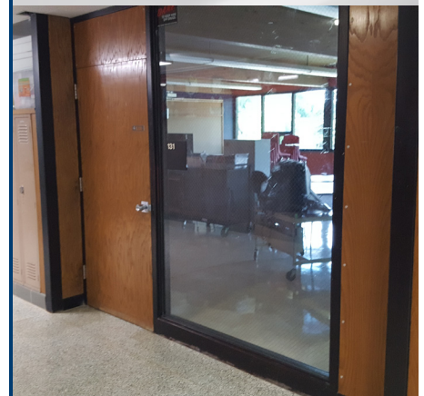
Noncompliant locksets with knob hardware in classroom doors
