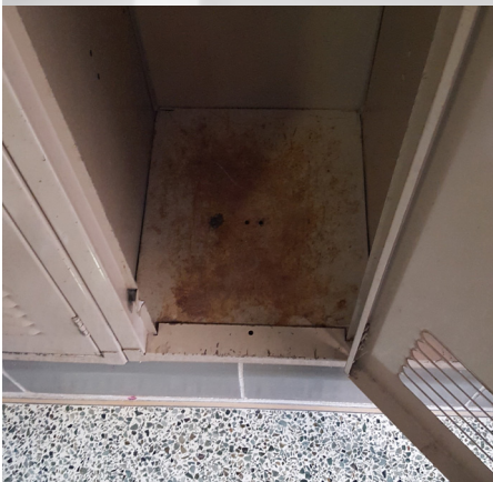
Damage and rusting in metal locker
