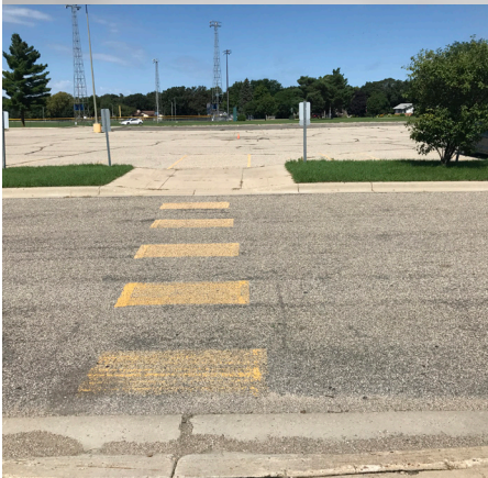
Faded crosswalk pavement markings in parking lot B's circulation areas
