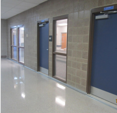
Doors and sidelights with wired glass
