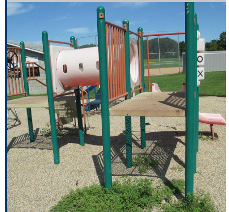
Rusted fasteners, warped platforms, faded paint, missing hardware in southernmost play unit
