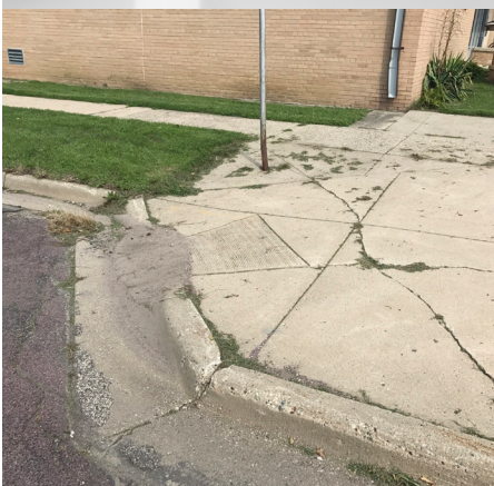
Cracking in concrete walkways
