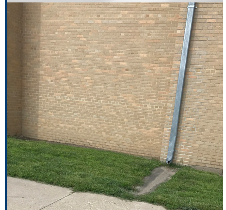
Damaged roof drains on the south face of the building
