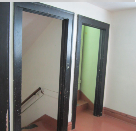
Noncompliant landings, and handrails on stairs
