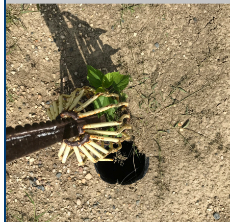
Uncovered field tile inlet
