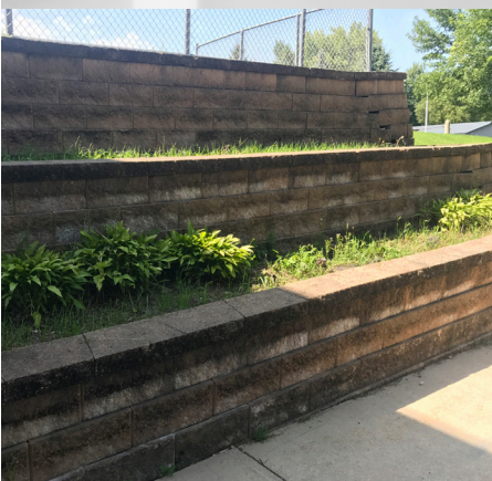
Stepped retaining walls
