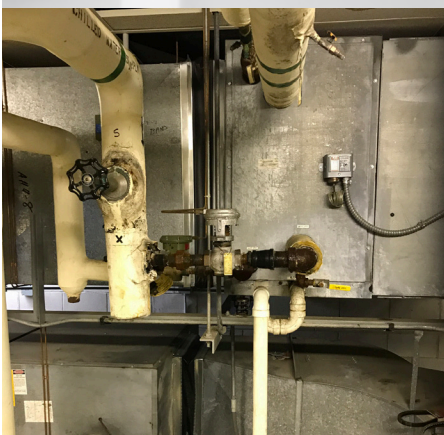
Uninsulated chilled water lines
