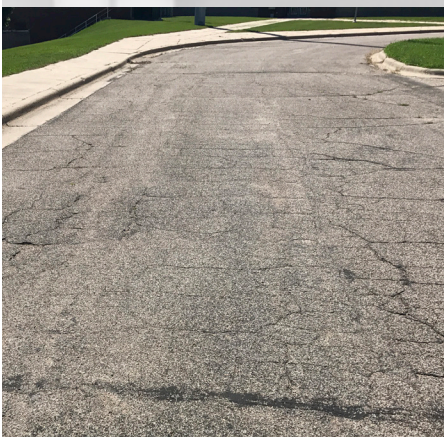
Alligator and block cracking along the northern portion parking lot B's circulation drive
