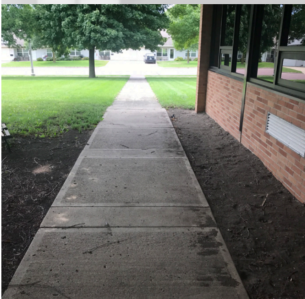
Discoloring, deflection of panels, cracking, and signs of weathering on concrete pavement
