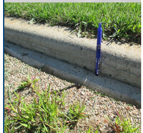
Weeds and loss of surfacing in landing pit
