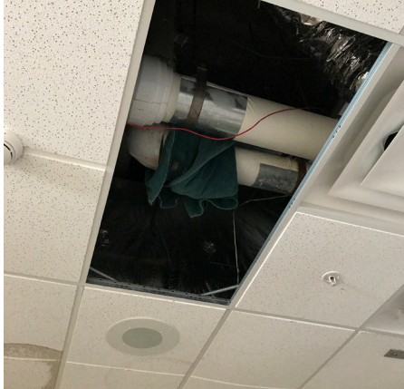
Damaged insulation
