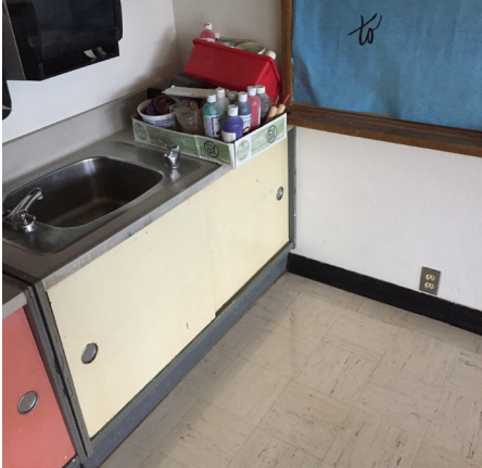
Receptacle near sink without GFCI protection
