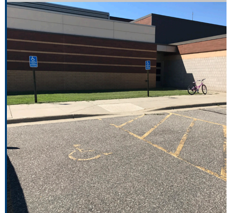
Faded pavement markings, no van accessible plaque at the van-accessible stall
