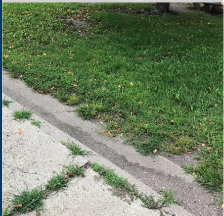
Sediment collection along gutter line on the north side of the pavement
