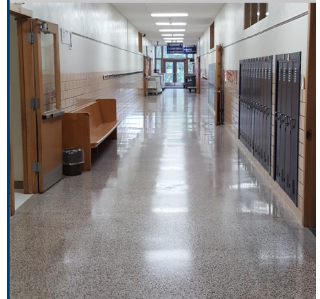
Glazed concrete block with painted plaster walls
