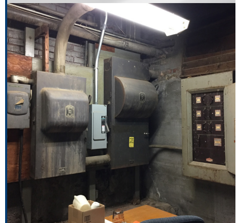
Original service main electrical gear
