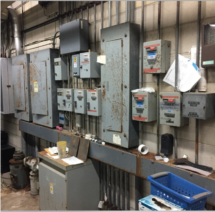
Rusted electrical equipment in pool mechanical room
