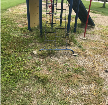
Exposed concrete footings of northwestern playground composite structure
