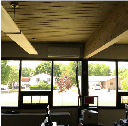
Mini split for cooling in computer lab
