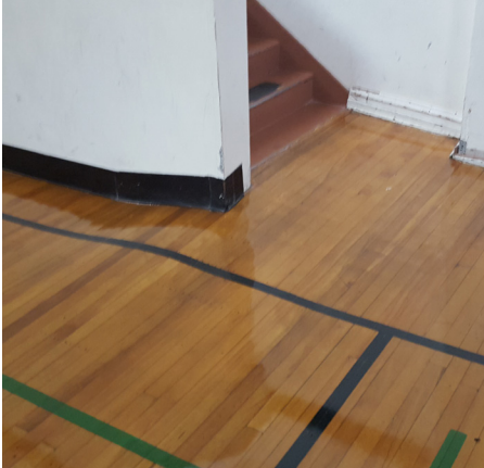
Wood floor with sloping at stairway
