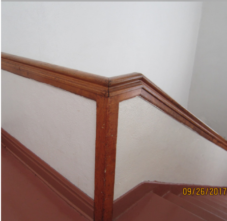
Noncompliant exit stairwell
