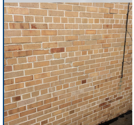
Stair step crack in brick façade
