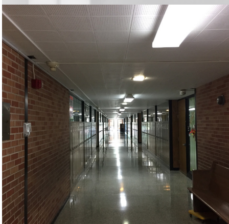
Corridor with a combination of fluorescent and incandescent lighting
