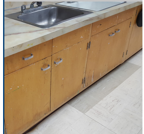
Damage and deterioration on casework
