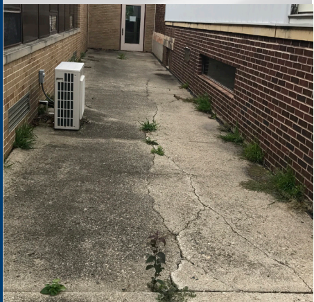
Cracking and discoloration of panels
