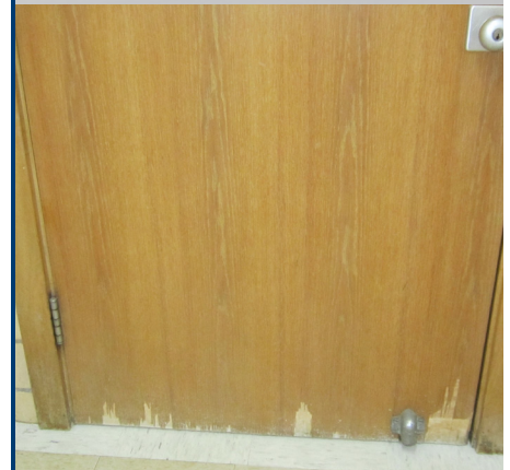
Damage and noncompliant knob hardware in wood doors
