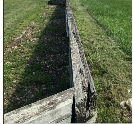
Rotting in wood retaining wall
