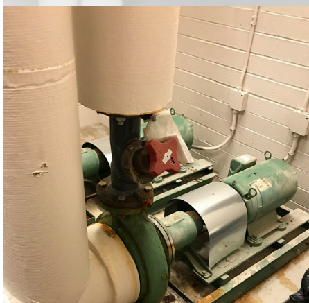
Uninsulated pipe and no vibration isolation
