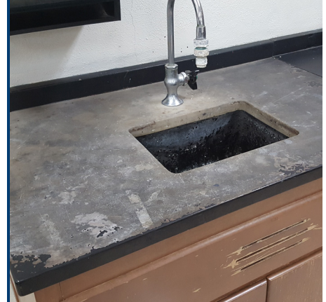
Damage and deterioration on casework
