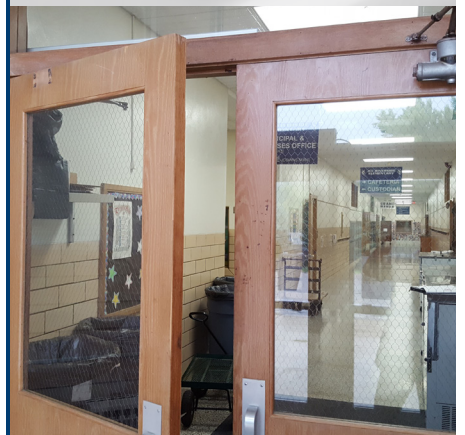
Noncompliant wired glass in doors and sidelights
