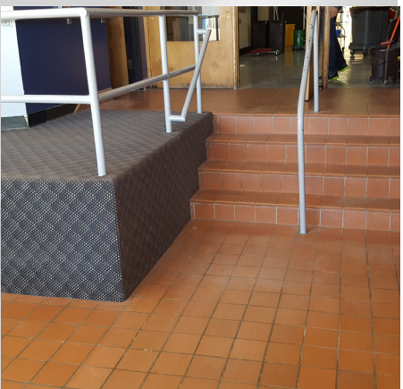
Noncompliant landings, handrails, guards and edge protection on ramps/stairs
