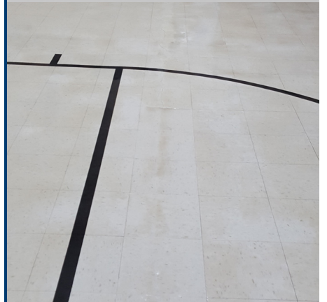
Cracking and discolored vinyl tile floor
