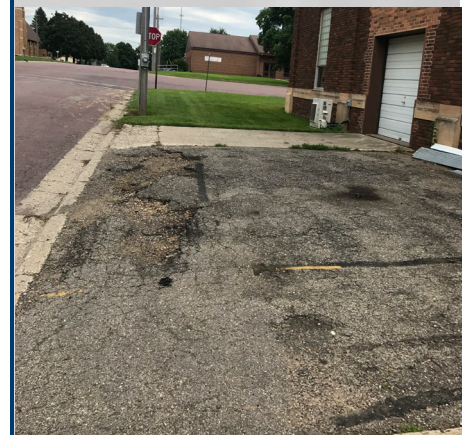
Damaged bituminous pavement separating concrete accesses
