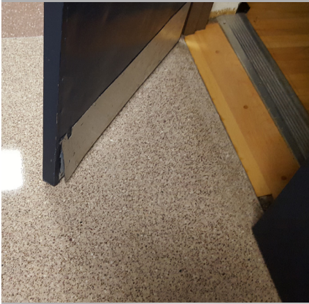
Door with dents and damaged kick plate
