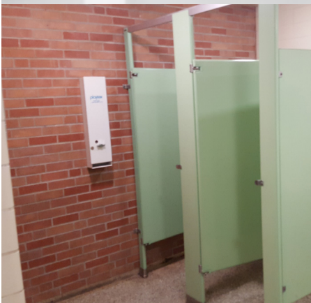
Missing wall base in restroom
