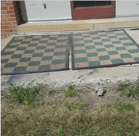
Door stoop height difference at exit doors
