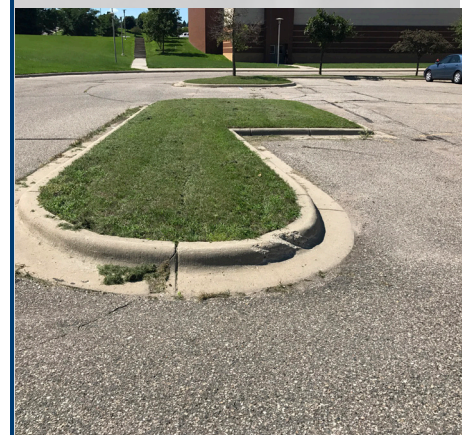
Cracking and scraping of the curb and gutter
