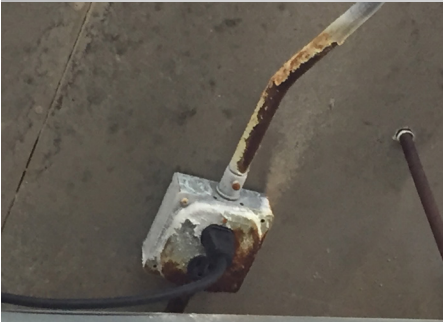
Rusted electrical equipment in pool mechanical room
