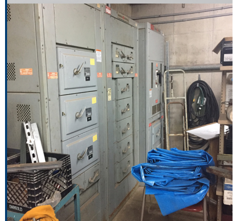
Main electrical gear without proper clearances
