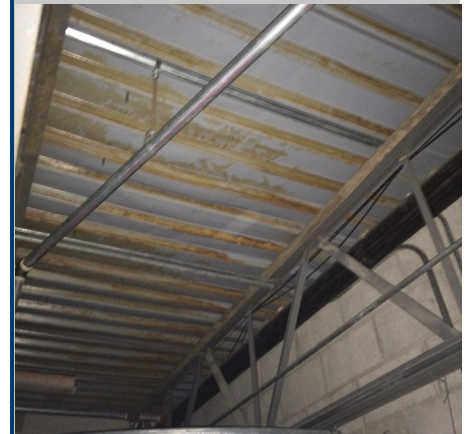
Rust on bottom of metal deck
