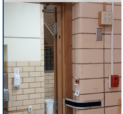
Damage and joint stain in glazed concrete block walls
