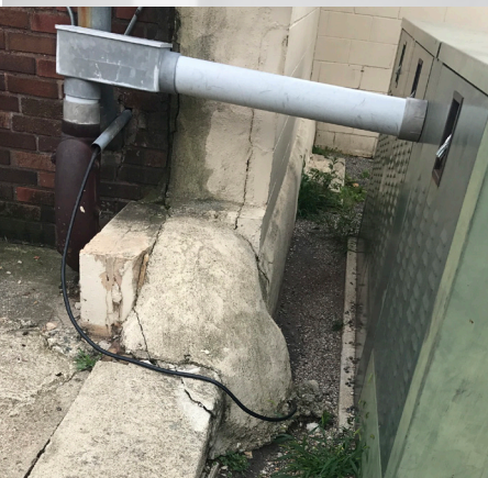
Utility cables cemented into the concrete edge.
