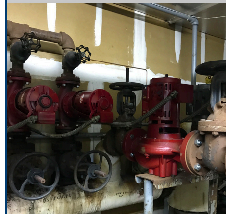
No vibration isolation on pump
