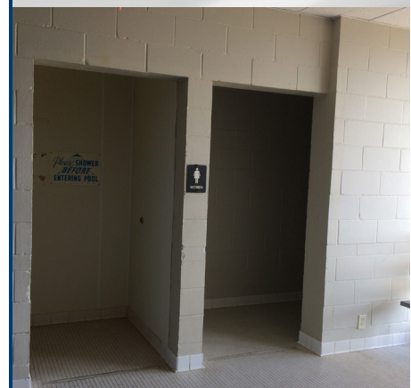
Noncompliant maneuvering clearances at entrance to restrooms and locker rooms
