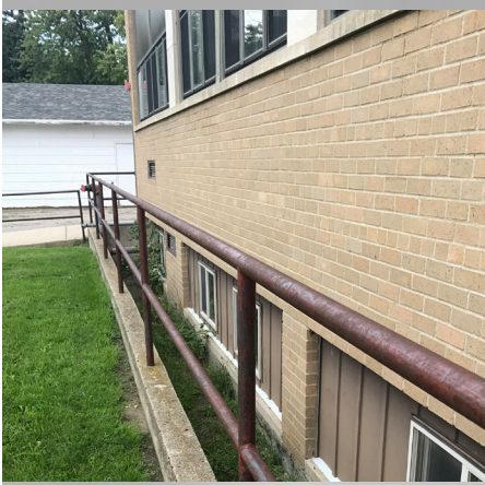
Rusted and sharp edges on railings
