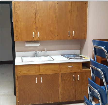
Sink with cabinets below, rather than clear floor space
