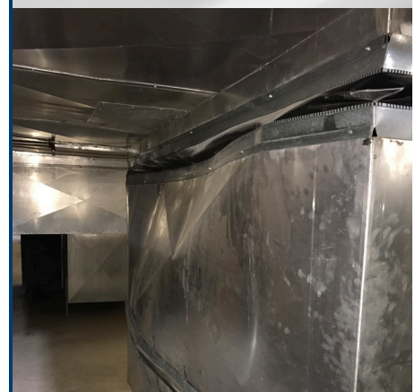
Bent and damaged ductwork
