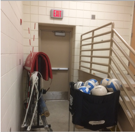
Partially blocked path to exterior exit door
