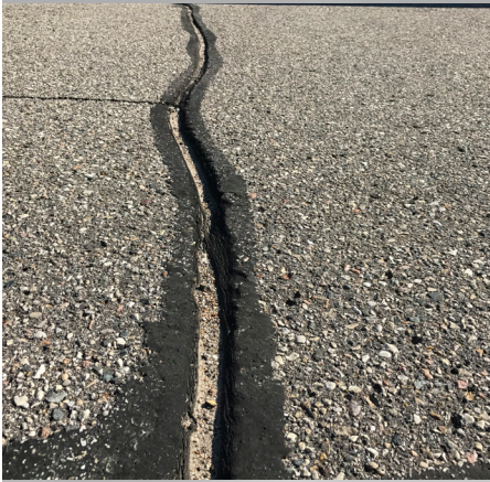
Previous joints losing seal in parking lot C
