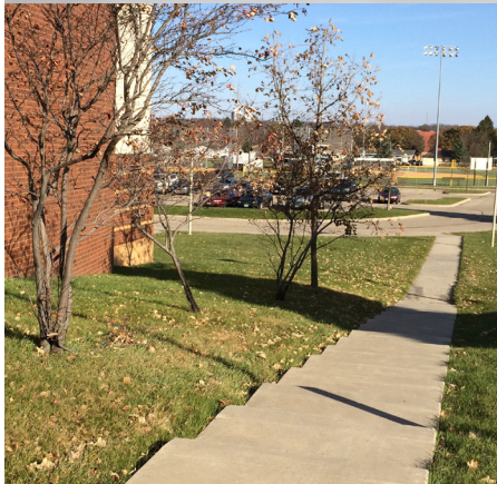
Lack of handrails on stairs
