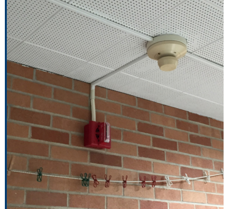
Typical fire alarm detection + notification devices
