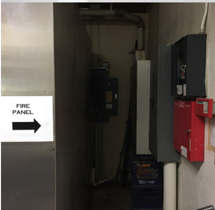
Fire alarm control panel with limited clearance
