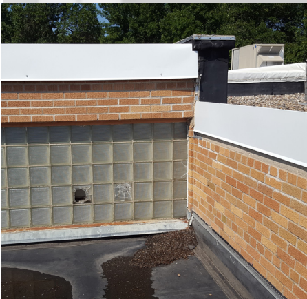
Damaged metal flashing and glass block at rubber roof
