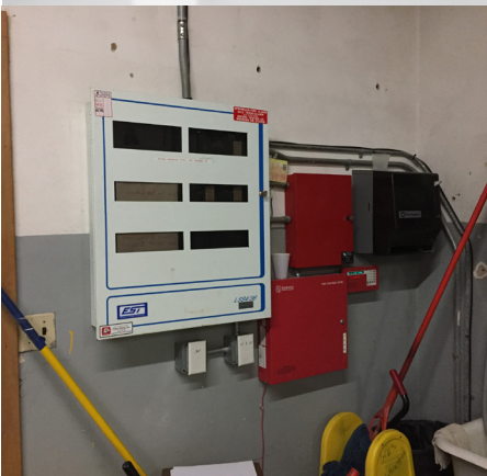
Fire alarm control panels
