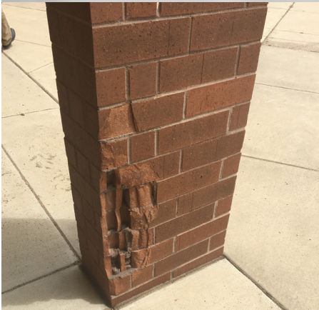
Brick column with damaged units
