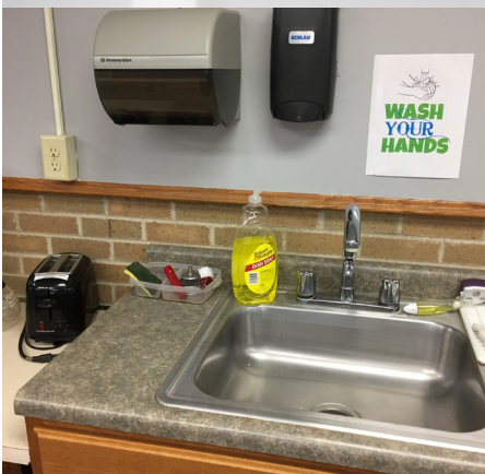
Non-GFCI receptacle near sink
