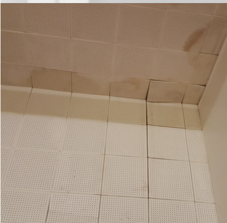
Stained, punctured, and cracked ceiling tiles
