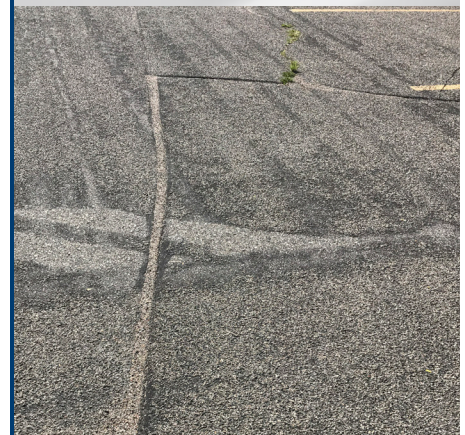
Exposed bituminous aggregate in parking lot A
