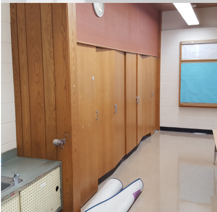
Damage in wood closet doors and trim
