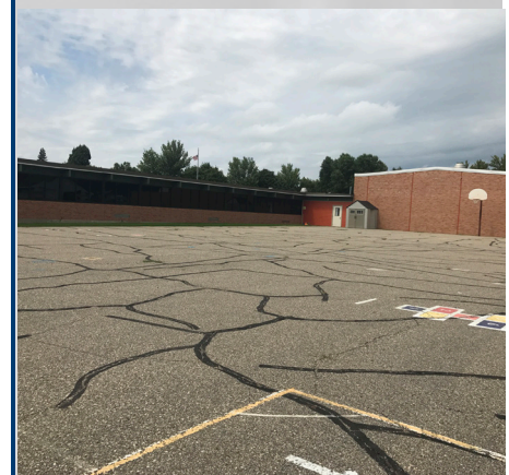
Crack filling and sealing of southern bituminous playground
