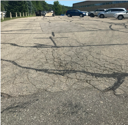
Alligator block cracking in north parking lot
