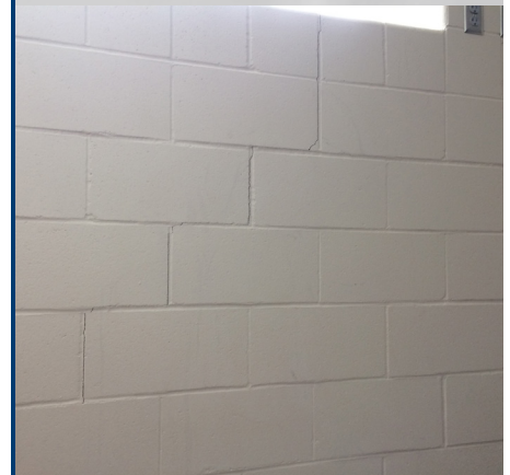
Stair step crack in CMU wall
