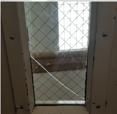
Damaged hollow metal door with wired glass
