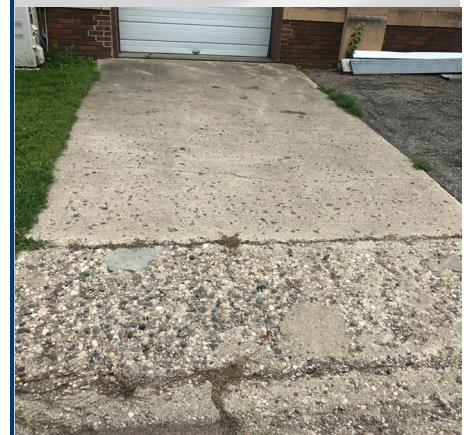
Cracking, exposed aggregate, vegetation, and signs of weathering on driveway
