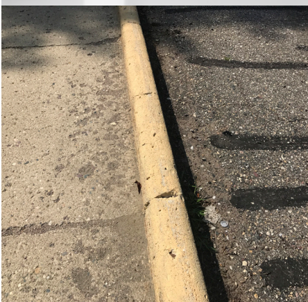
Minor cracking and faded paint on curb
