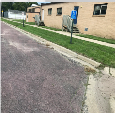
Sediment collection at the junction of the sidewalk panels and curb line
