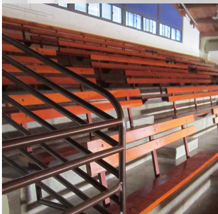
Noncompliant egress, stairways, handrails and guards; no accessible seating.
