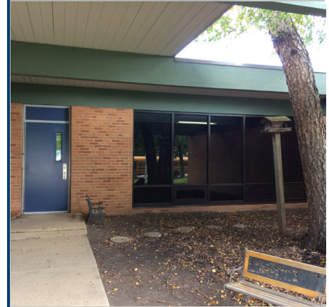
Height difference in stoop and door sill in courtyard entrance
