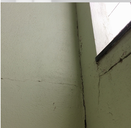
Plaster Cracks in east wing
