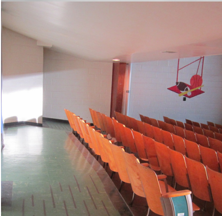
Nonslip striping and slopes in all directions on floor tile
