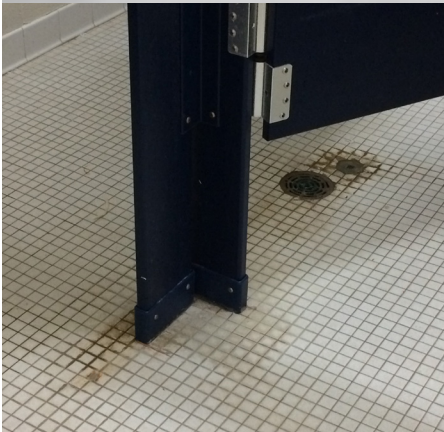
Restroom tile floors stained and cracking
