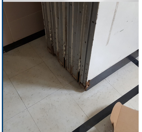
Edge chipping and marks where items were previously attached in room divider panels
