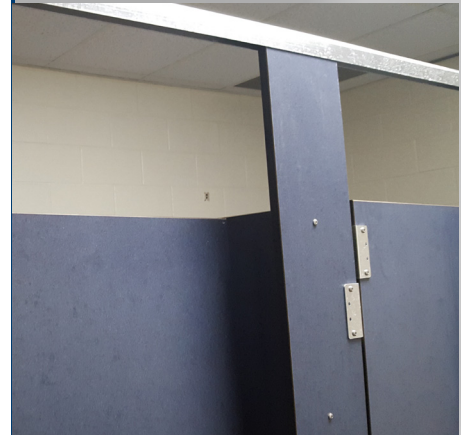
Restroom toilet partitions with damage and rusting
