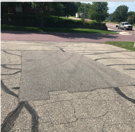
Crack filling, seal coating and patching
