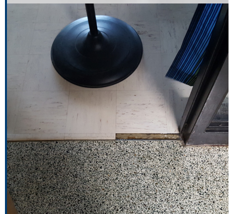
Cracking and missing tile floor at door
