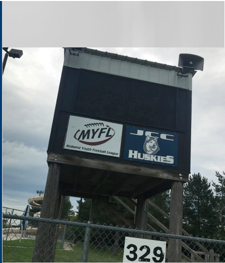
Weathered wood and cracking in press box support posts
