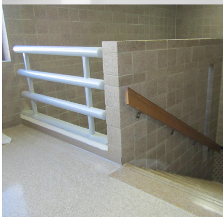
Noncompliant handrails and guards
