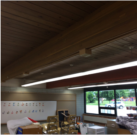
Glue-laminated Beams
