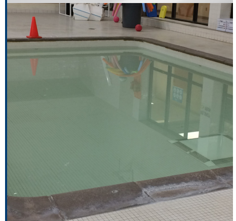
Surface corrosion around wading pool
