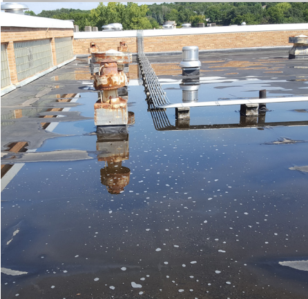
Large amount of standing water on rubber roof
