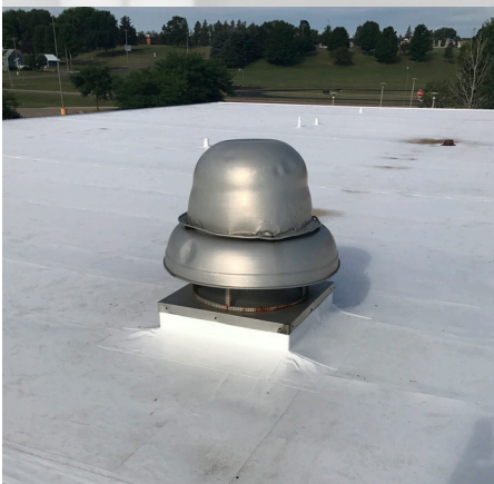
Exhaust fan in need of replacement
