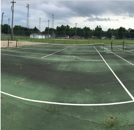
Areas of settlement, discoloration, and cracking in tennis court
