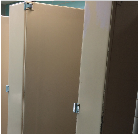
Chipped and rusting at seams in toilet partitions
