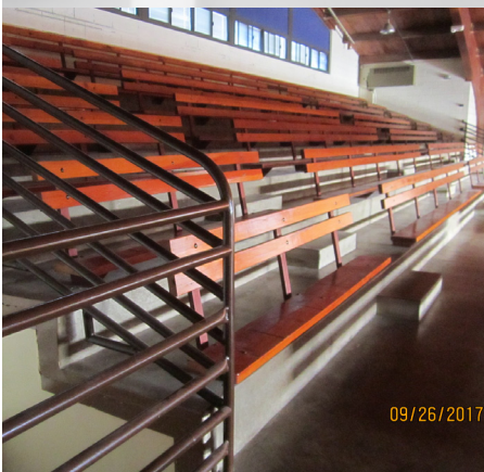
Non existing second means of egress from balcony
