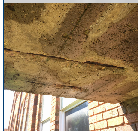
Exposed rebar at stairs
