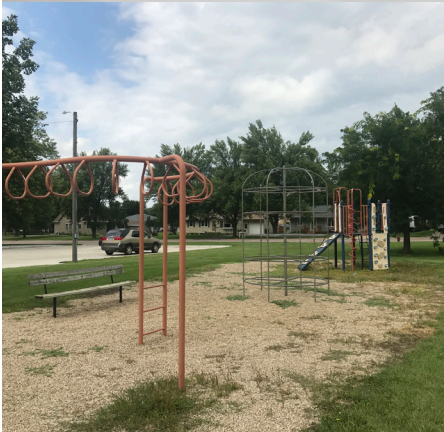
Rusted metal climbing structure in northwest play area and faded paint on overhead loop ladder
