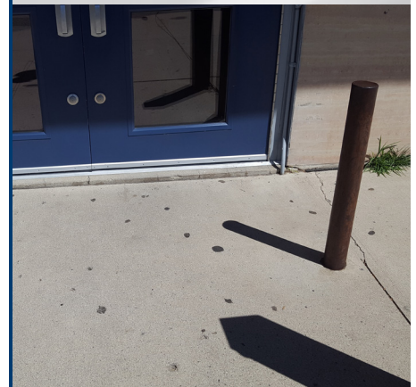
Elevation differences in stoops and sidewalks in exterior doors
