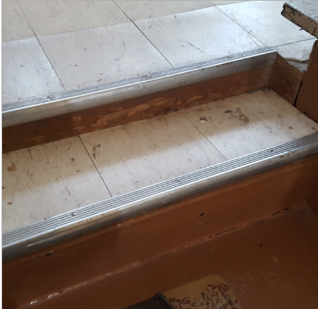
Noncompliant risers and treads on stairs
