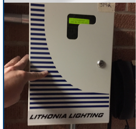
Lighting control panel for gymnasium
