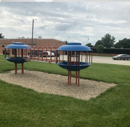
Hazards in piece of playground equipment presenting areas of entrapment and short safety zone
