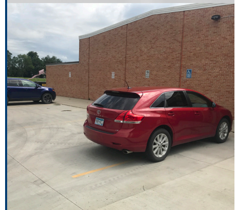
Handicap spaces not striped with an access aisle or pavement symbol
