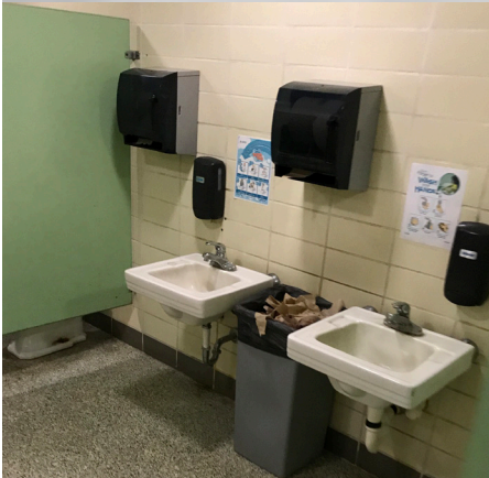
Pipe wrap missing below lavatories
