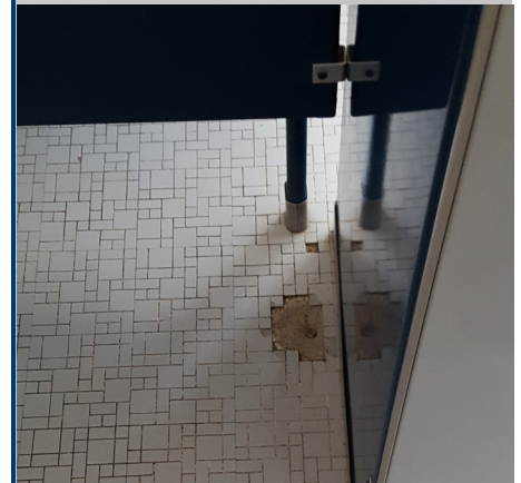
Stained, missing tile in restroom floor
