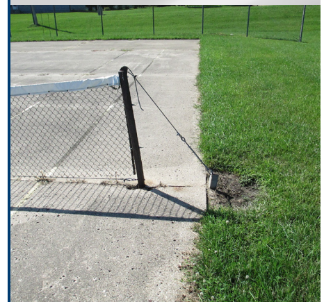
Rusted net posts and connections
