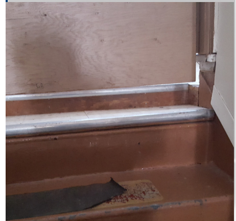
Damaged slip resistance materials; no stairway landing
