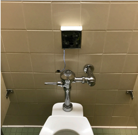
Replaced flush valve with exposed wire
