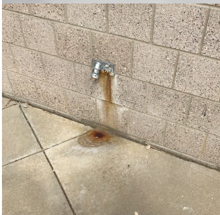
Leaking exterior hose bib
