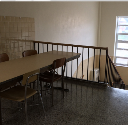
Noncompliant handrails and guards on stairways
