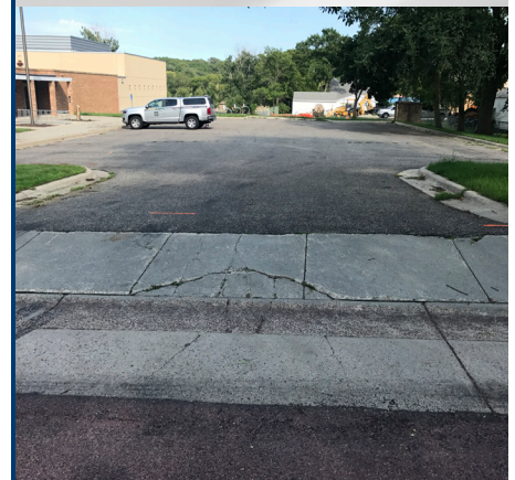
Cracking in concrete pavement of the southern parking lot driveway apron
