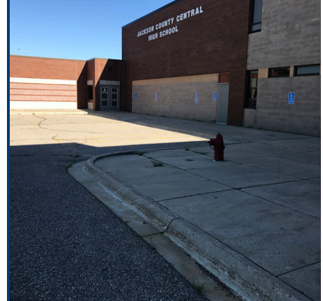
Sidewalk settling below curb
