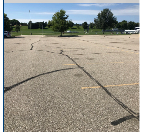
Cracks and potholes have formed and previous joints beginning to lose their seal in parking lot B
