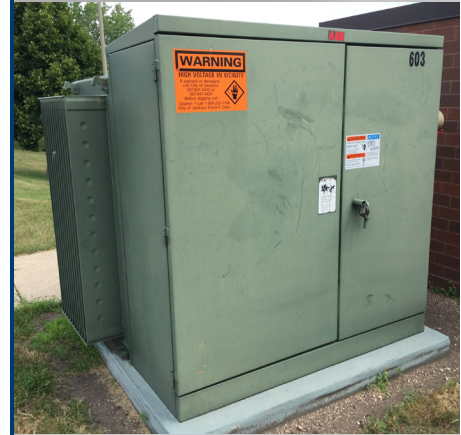
Electrical utility transformer
