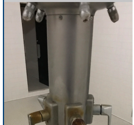
Leaking shower fixtures
