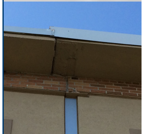
Missing Mortar in Stone at Joint
