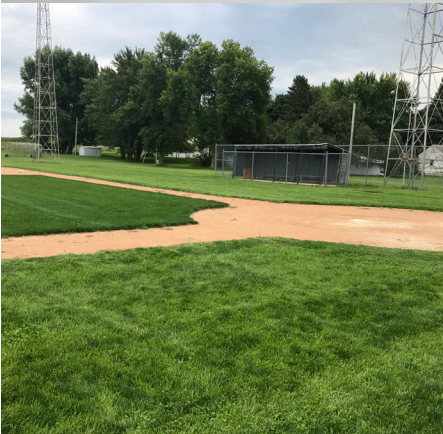
Aglime surfacing loss near grass edges
