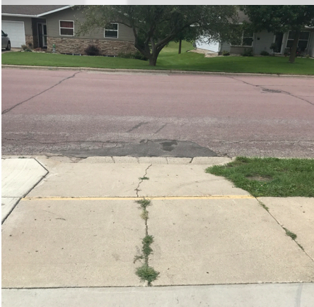
Cracks in the gutter line pavement in accessible ramp leading to main school doors
