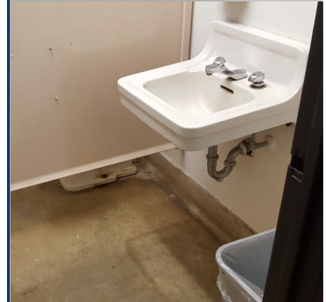
Stained sealed concrete floor around sink and toilet
