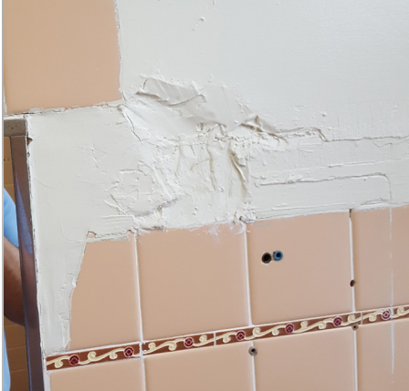
Damage to plaster restroom walls
