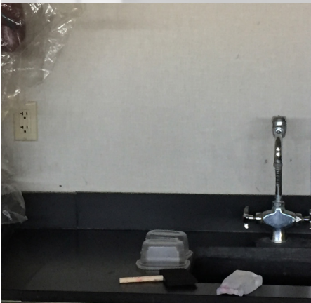
Non-GFCI receptacle near sink
