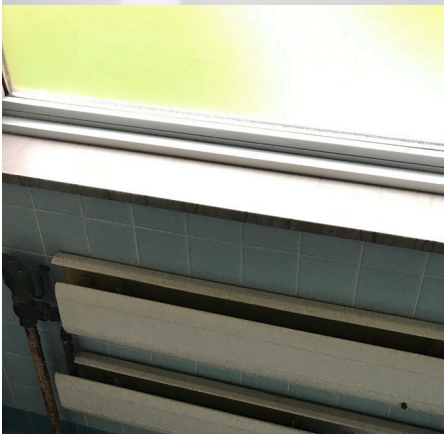
Fin tube cover is missing
