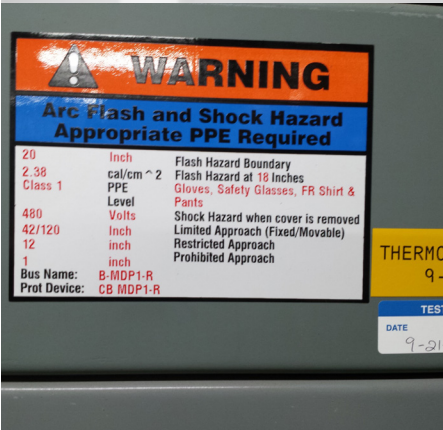
Typical Arc Flash Hazard label required by NEC
