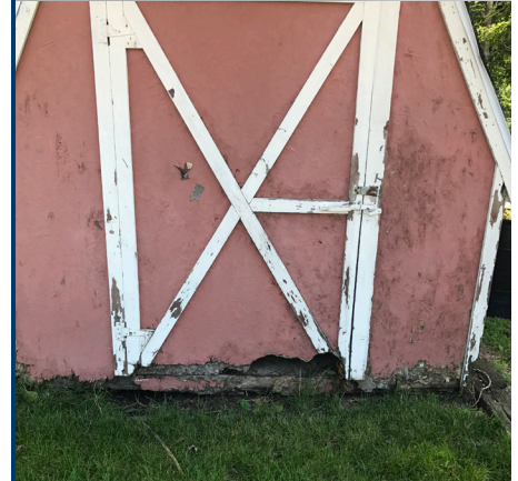
Rotten wood with missing shingles in storage shed on south side of the south baseball field
