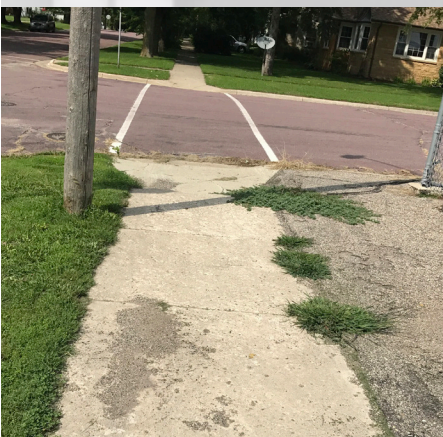
No advance detectable warning tiles on walkway accessible ramps and sediment collection
