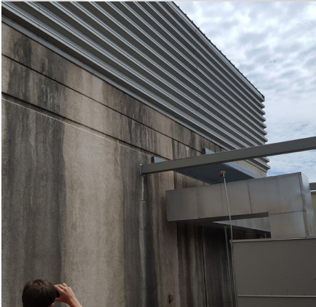
Stucco wall with severe staining and mold
