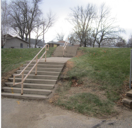
Cracking and a handrail in the center rather than on the sides on concrete stairway
