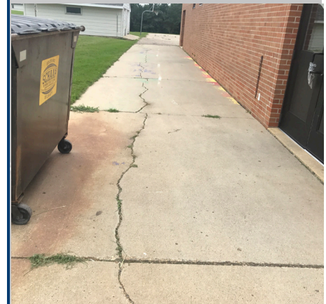
Cracking and discoloring in eastern sidewalk
