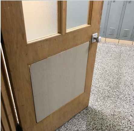
Transfer grille in door is covered
