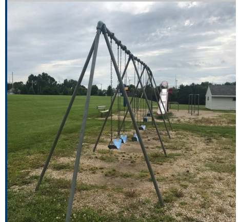
No rubber chain, mounted on discolored scraped metal frame
