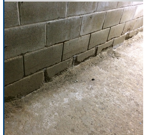
Deteriorating CMU wall in basement
