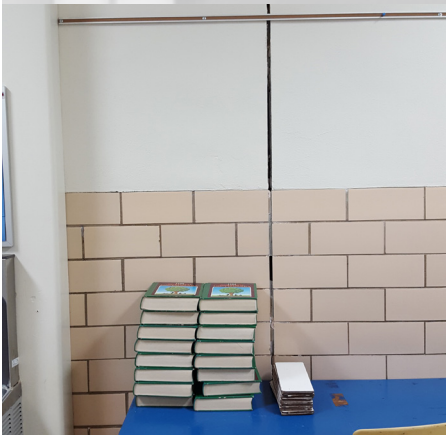
Damage in glazed concrete block walls, cracking in plaster above
