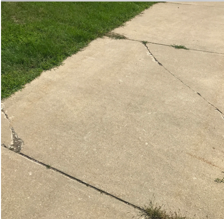
Corner breaking on five of the north walkway panels
