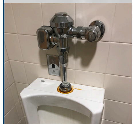
Stained fixture due to leaking flush valve
