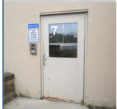
Rusting, peeling paint and damage on metal door
