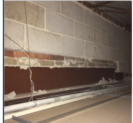
Missing CMU above steel beam
