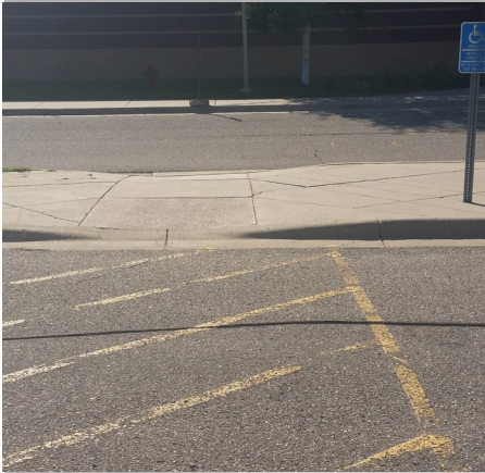
Noncompliant curb ramps and pedestrian crosswalk
