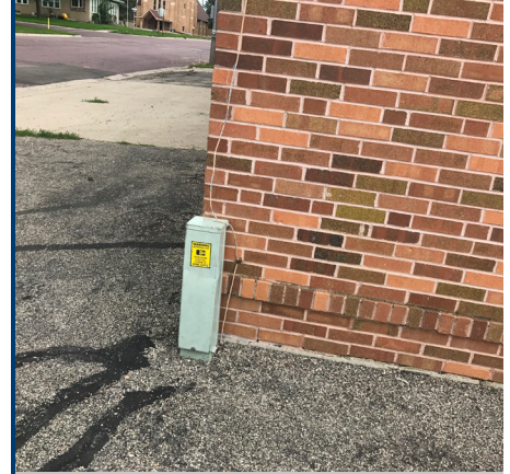
Worn and warped electrical pedestals covers
