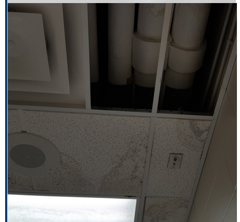
Ceiling with moisture damage
