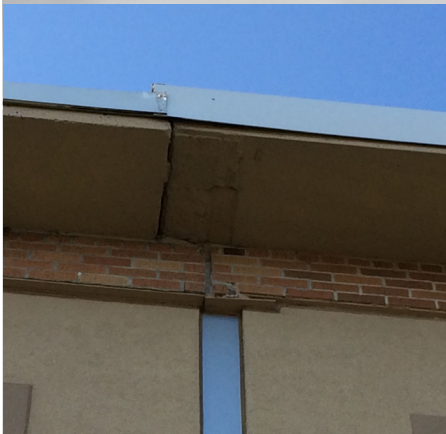
Missing mortar in stone at joint
