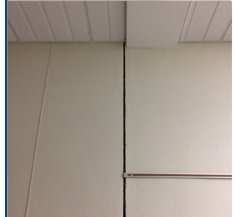
Missing sealant in joint
