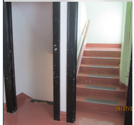
Noncompliant landings in exit stairways
