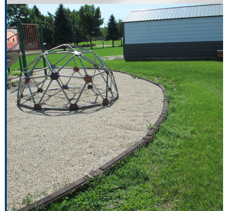
Rusted connections points in geodesic dome climber
