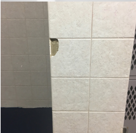
Cracked tile in restroom
