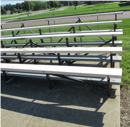
Rusting and missing end caps in bleachers
