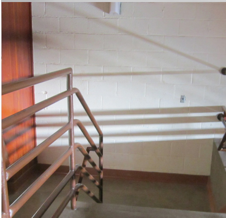
Noncompliant handrails and guards on stairs
