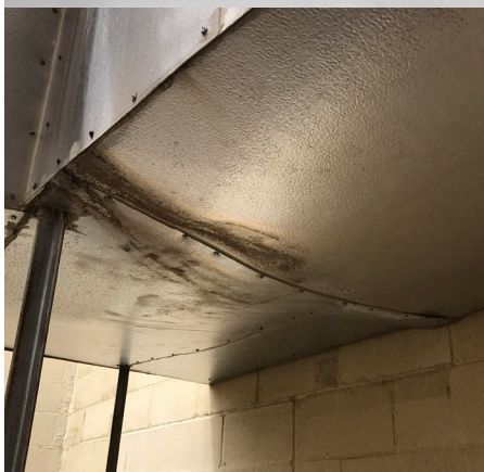
Damaged exterior insulation with standing water inside
