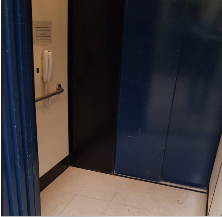
Limited maneuvering clearances in elevator cab
