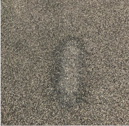
Exposed aggregate on bituminous pavement of parking lot B
