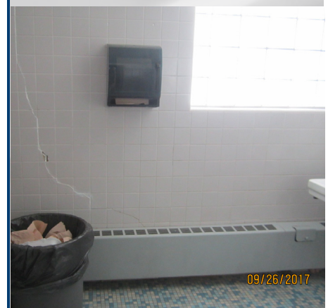
Cracking wall tiles
