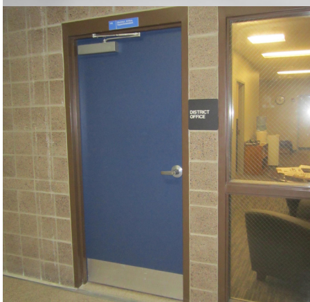
Noncompliant wired glass in sidelight
