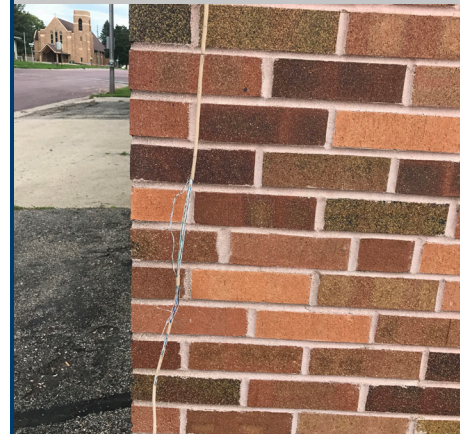
Lack of protective coating and fraying on cables
