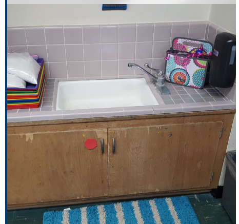
Damage in cabinet and sink casework
