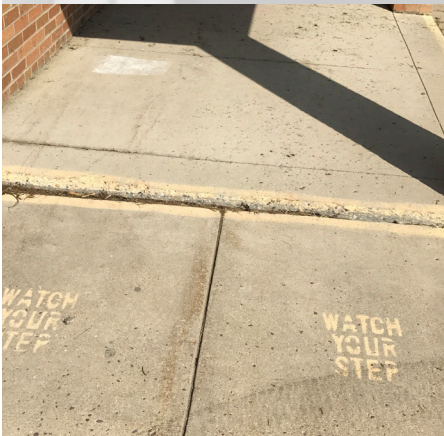
Concrete pavement raised approximately 2-3 inches from adjacent sidewalk
