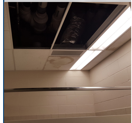
Damaged ceiling tiles
