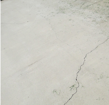
Cracks in pole vault concrete pad
