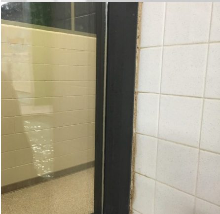
Degraded sealant joints in pool area
