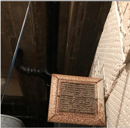
Dirty and rusted exhaust grilles
