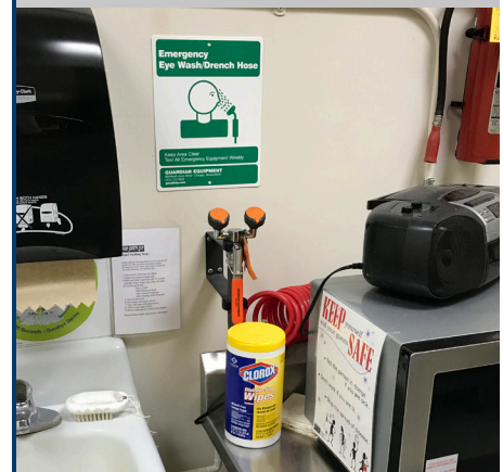
Eyewash station with no thermostatic mixing valve
