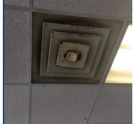
Rusted diffuser in pool area
