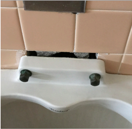
Fixtures Loose from Wall
