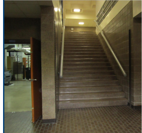
Handrails not extended properly at bottom and tops of stairwell
