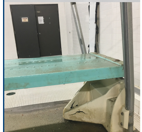
Corrosion on diving board attachment to concrete base
