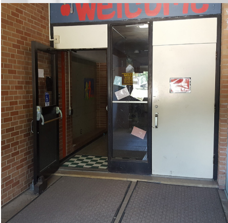
Vestibule floor at entrance is lower than corridor floor
