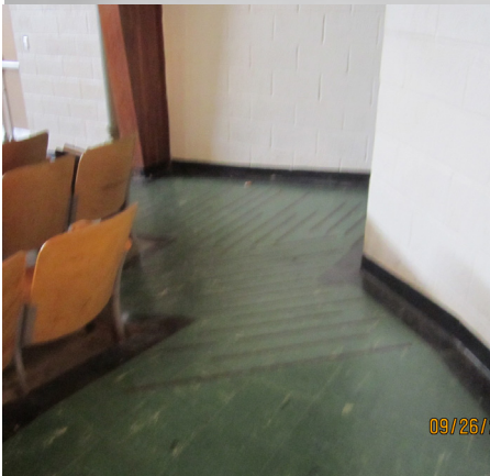
Noncompliant floor slope
