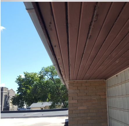
Rusting and peeling on soffits and trim
