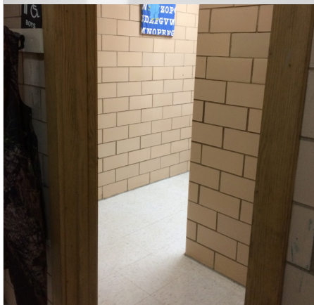
Glazed concrete block wall in basement
