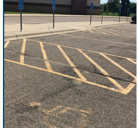
Faded pavement markings in parking lot A
