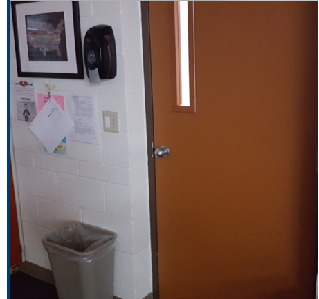
Noncompliant knob hardware and vision panel
