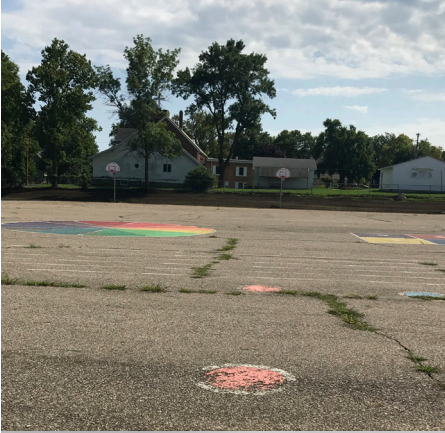
Cracks and localized depressions throughout bituminous play area pavement
