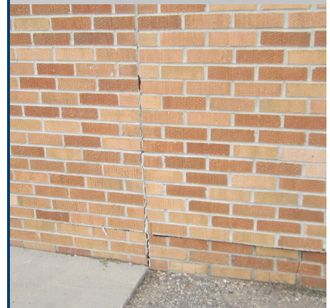
Cracking and joint failure, and discoloration on brick wall
