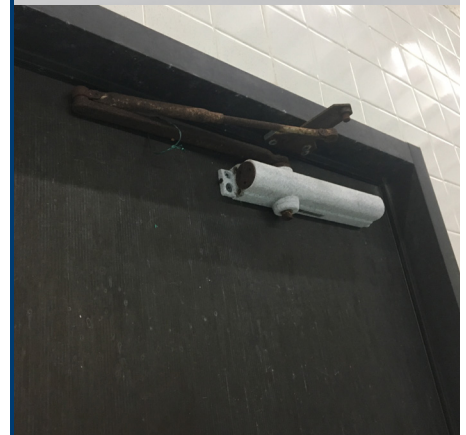
Rusted, damaged door in pool area
