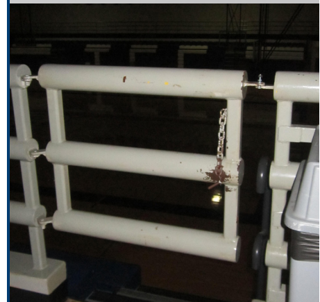
Noncompliant guard opening limitation
