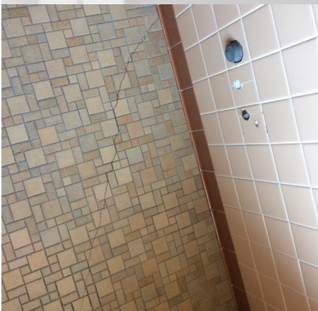
Crack in floor of boys' restroom
