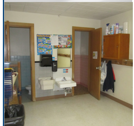
Limited maneuvering clearance on the pull side on the restroom doors
