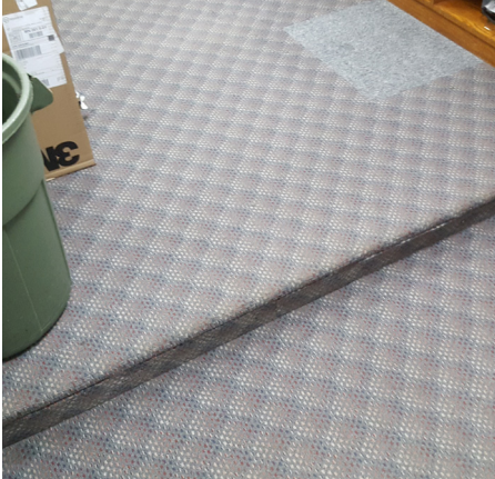
Noncompliant elevation change
