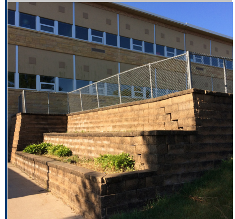
Damaged retaining wall
