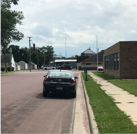
Lack of pavement markings/stripping and designating parking spaces.
