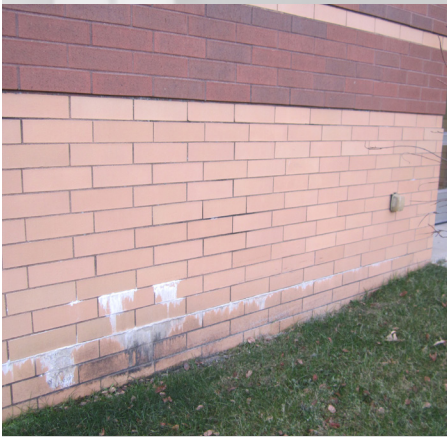
Brick wall with significant efflorescence
