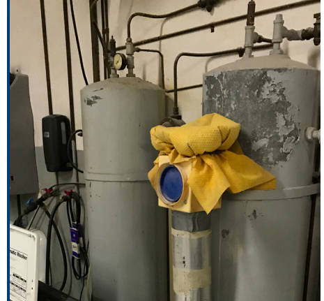
Dryer vent should be ducted to exterior
