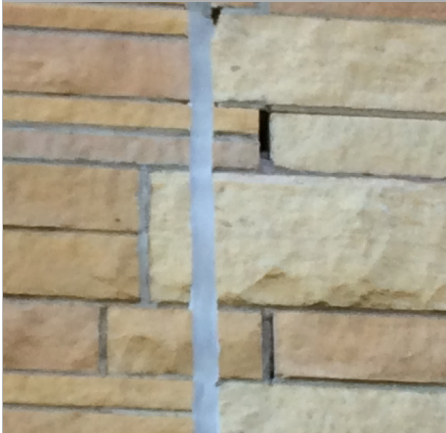
Missing mortar in stone at joint
