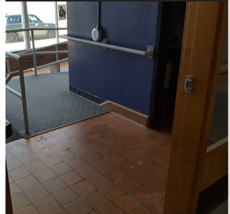
Uneven and noncompliant guards at entrance
