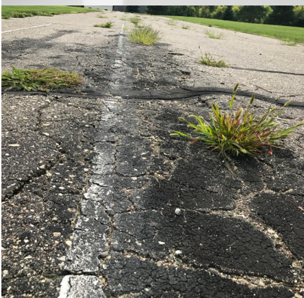
Severe cracking and vegetative growth within the bituminous surfacing
