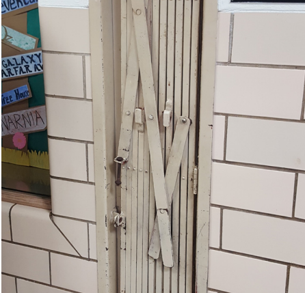
Recessed folding metal scissor gates
