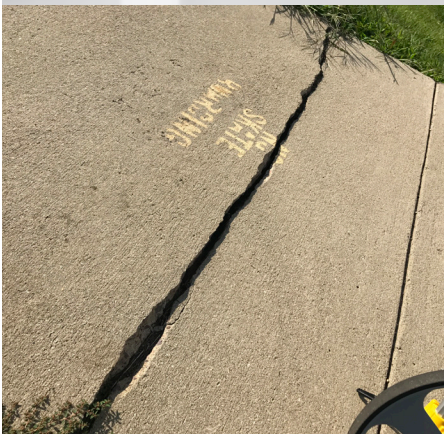
Cracking on the landings of stairs connecting the southern parking lot to the bituminous play area
