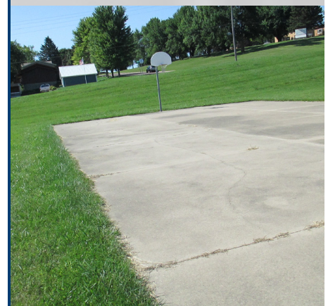
Discoloration and cracking throughout the pavement panels in basketball court
