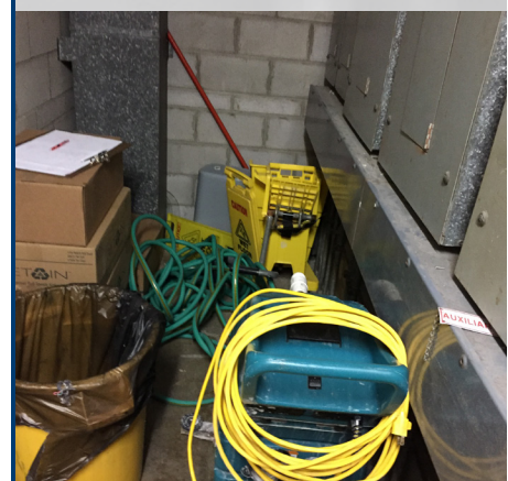
Branch panels without proper clearances
