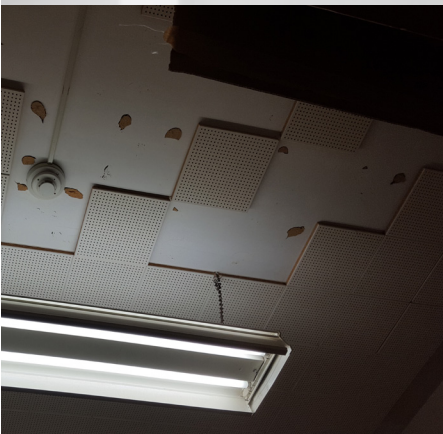
Uneven and missing ceiling tiles
