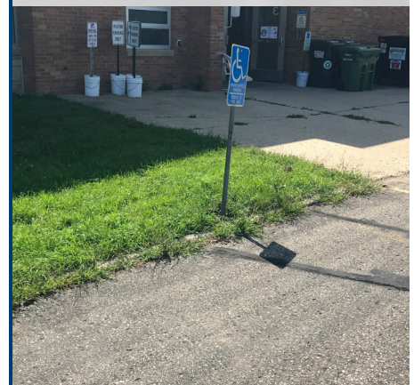
Handicap parking sign below the ADA 60 inch height requirement
