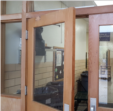
Wired glass in corridor door systems and sidelights
