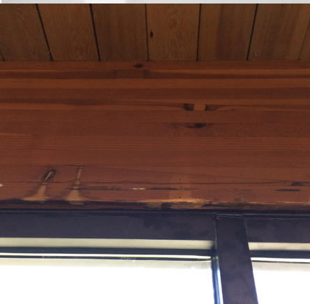
Moisture damaged glue-laminated beams
