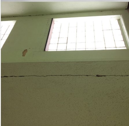
Plaster cracks in east wing
