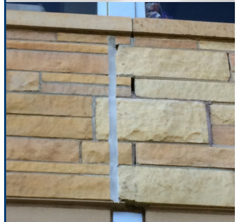
Missing Mortar in Stone at Joint
