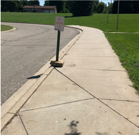
Sign not properly mounted within the adjacent concrete sidewalk pavement
