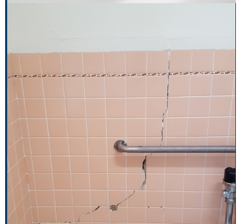
Cracking in ceramic tile with damage above in plaster wall
