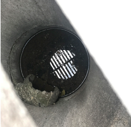
Cracking on chamber of reinforced concrete
