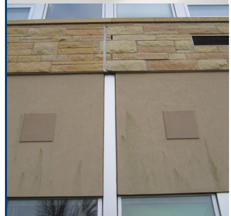
Discoloration and peeling at corners on stucco panels
