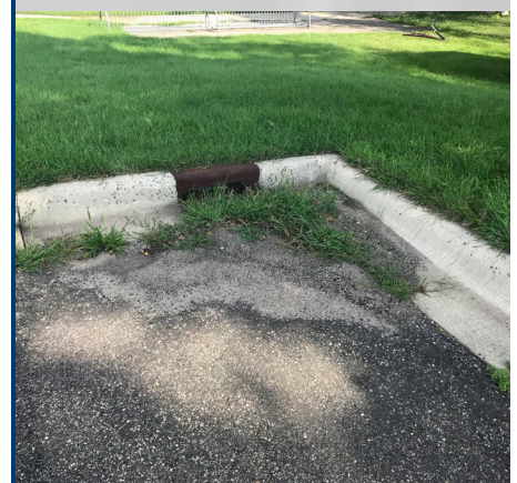
Sediment and vegetation buildup in front of south parking lot catch basin
