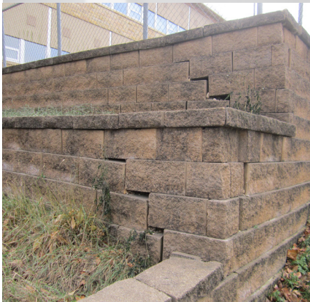
Shifting at corners of stone retaining walls
