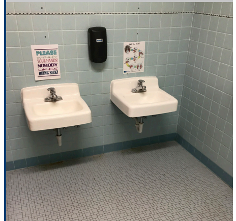
Pipe wrap missing below lavatories
