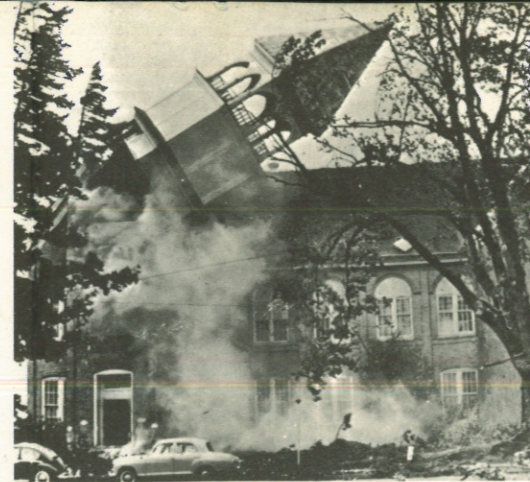
Philharmonic Hall, first unit of New York's projected Lincoln Center for Performing Arts, opened in a blaze of light. Steeple at Oregon State College of Education, Monmouth, Oregon, fell before hurricane-force winds which raked the West Coast in October causing major damage and communication breakdown.
