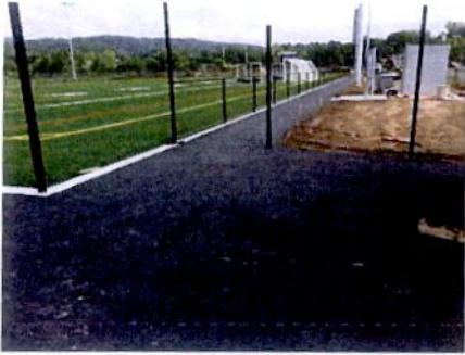
New asphalt put down to provide ADA access to new turf and existing grass fields.
