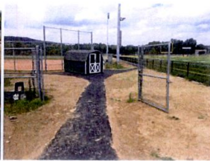
New asphalt put down to provide ADA access to new turf and existing grass fields.
