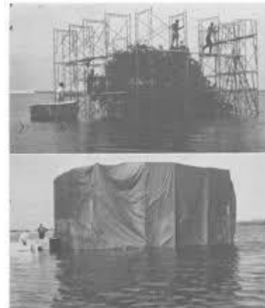
FIG. 8. Upper: The scaffolding constructed around E7, complete except for the top walkway. Lower: the fumigation tent over E7.
