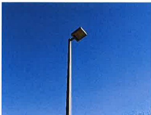
FIGURE 72 – SINGLE-POLE METAL HALIDE FIXTURE
