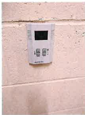
FIGURE 50 – TYPICAL DDC THERMOSTAT
