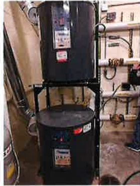
FIGURE 75 – INSTANTANEOUS WATER HEATERS
