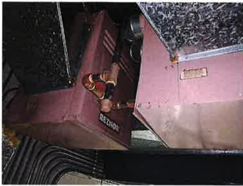
FIGURE 47 – WEIGHT ROOM DUCT FURNACE
