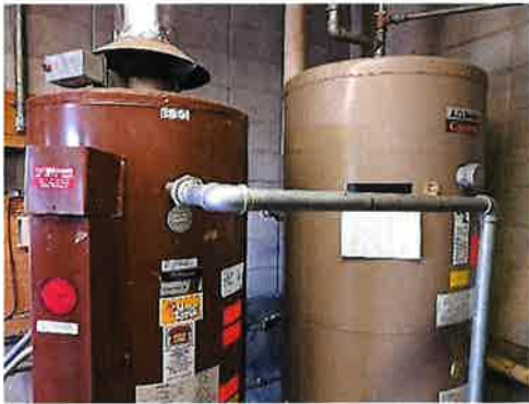
FIGURE 82 – GYM DOMESTIC HOT WATER SYSTEM
