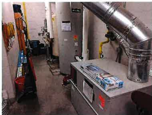
FIGURE 77 – DOMESTIC HOT WATER SYSTEM #1
