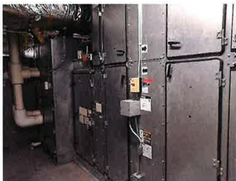
FIGURE 24 – HOT DECK AIR HANDLER
