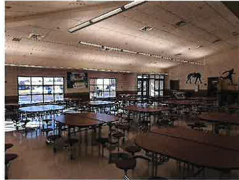
FIGURE 60 – TYPICAL T8 DIRECT/INDIRECT FIXTURES
