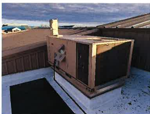
FIGURE 40 – 5-TON RTU
