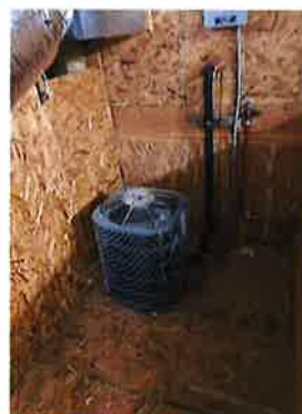
FIGURE 28 – SERVER ROOM CONDENSING UNIT
