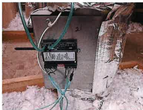
FIGURE 53 – TYPICAL DDC CONTROLLER
