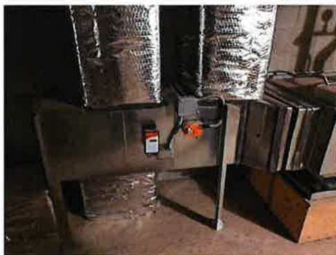
FIGURE 18 – DUCT MOUNTED CO2 SENSOR
