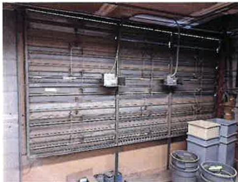
FIGURE 44 – GYM AHU OUTSIDE AIR LOUVER
