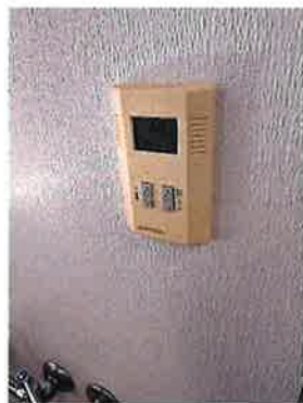
FIGURE 52 – TYPICAL DDC THERMOSTAT
