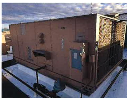
FIGURE 41 – 20-TON RTU
