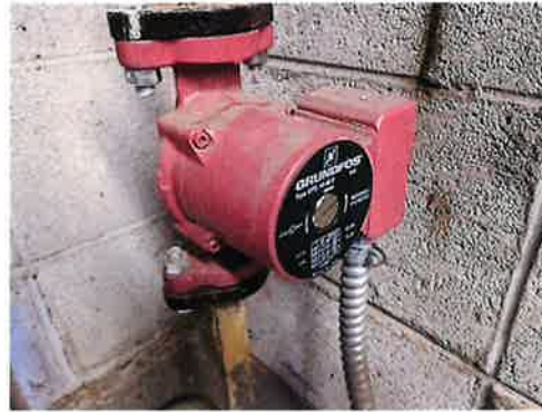
FIGURE 83 – GYM RECIRCULATION PUMP
