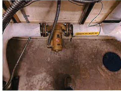
FIGURE 76 – DOMESTIC HOT WATER RECIRCULATION PUMP
