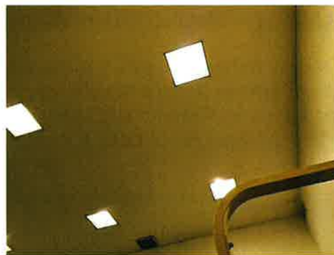
FIGURE 66 – WEIGHT ROOM METAL HALIDE FIXTURES
