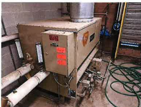
FIGURE 33 – HOT WATER BOILER
