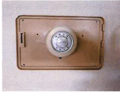
FIGURE 56 – TYPICAL NON-PROGRAMMABLE THERMOSTAT
