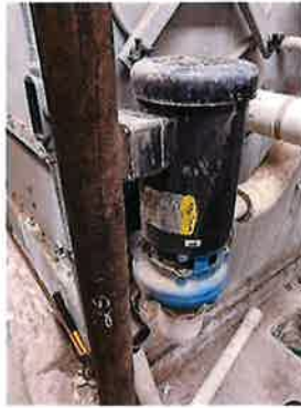
FIGURE 37 – COOLING TOWER PUMP
