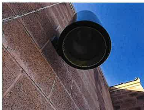
FIGURE 73 – CYLINDER METAL HALIDE FIXTURE
