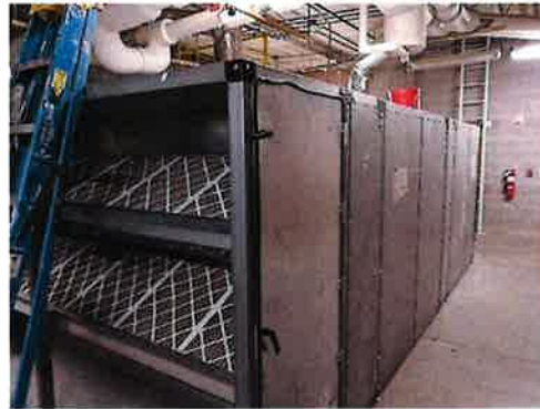
FIGURE 23 – COLD DECK AIR HANDLER
