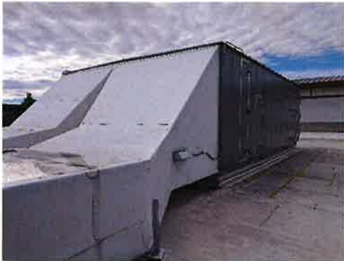
FIGURE 19 – ENERGY RECOVERY UNIT
