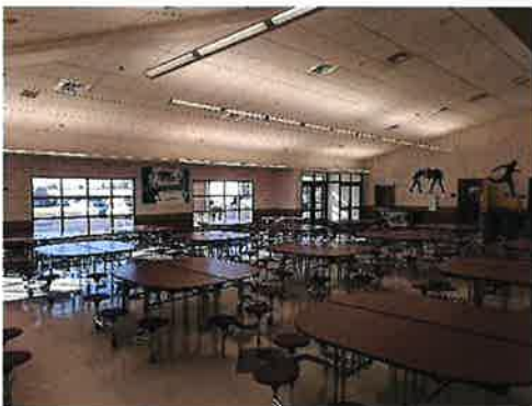
FIGURE 61 –TYPICAL T8 ACRYLIC FIXTURES
