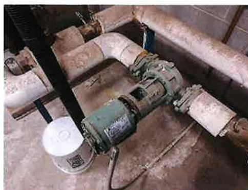
FIGURE 34 – HOT WATER BOILER PUMP
