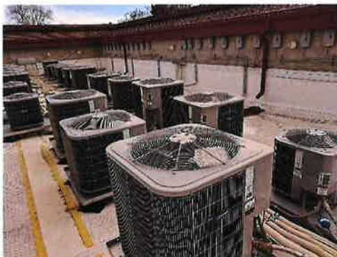
FIGURE 16 – ROOF-MOUNTED CONDENSING UNITS
