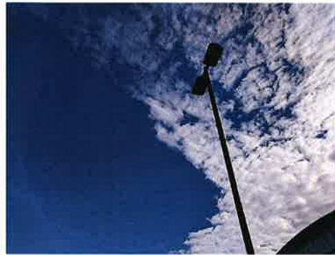
FIGURE 68 – DOUBLE-POLE METAL HALIDE FIXTURE
