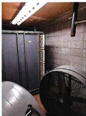
FIGURE 45 – GYM AHU RETURN AIR OPENING
