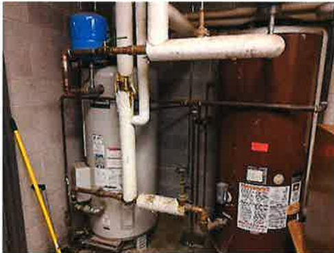
FIGURE 80 – DOMESTIC HOT WATER SYSTEM
