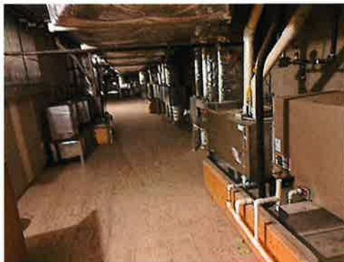
FIGURE 17 – FURNACES LOCATED IN ATTIC
