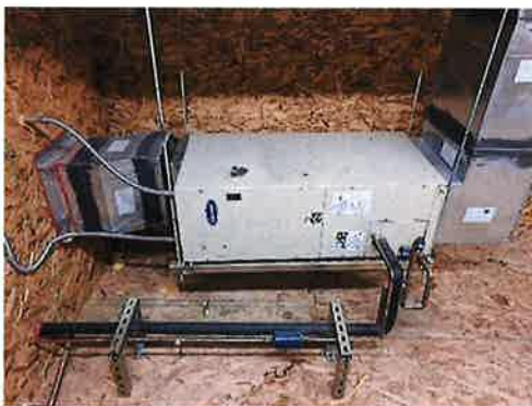
FIGURE 27 – SERVER ROOM FAN COIL UNIT
