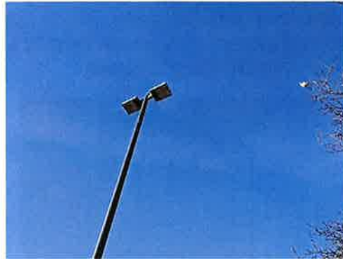
FIGURE 70 – DOUBLE-POLE METAL HALIDE FIXTURE
