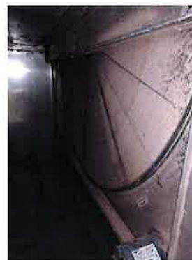
FIGURE 25 – HEAT RECOVERY WHEEL
