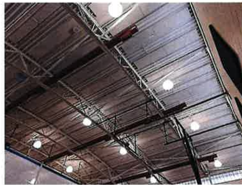
FIGURE 58 – GYMNASIUM METAL HALIDE FIXTURES
