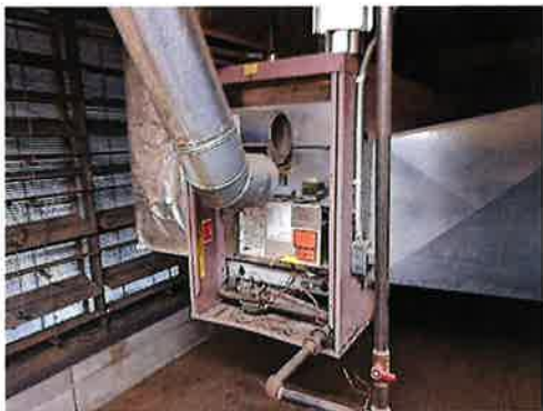
FIGURE 43 – GYM AHU DUCT FURNACE
