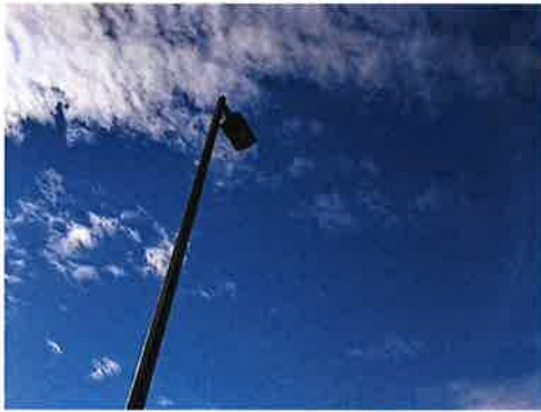
FIGURE 67 – SINGLE POLE METAL HALIDE FIXTURE
