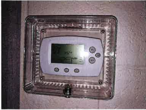
FIGURE 55 – TYPICAL PROGRAMMABLE THERMOSTAT
