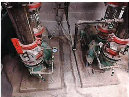
FIGURE 35 – CONDENSER LOOP PUMPS
