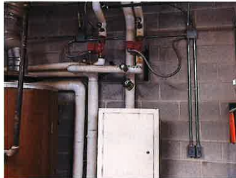
FIGURE 81 – RECIRCULATION PUMP
