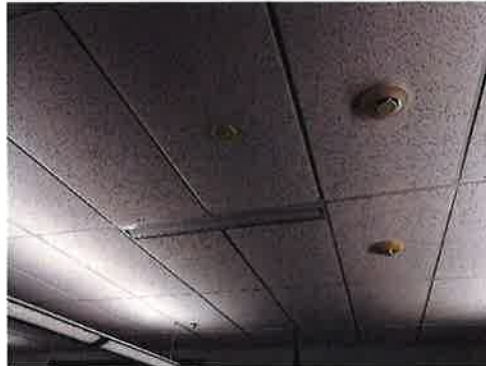
FIGURE 54 – TYPICAL OCCUPANCY SENSOR
