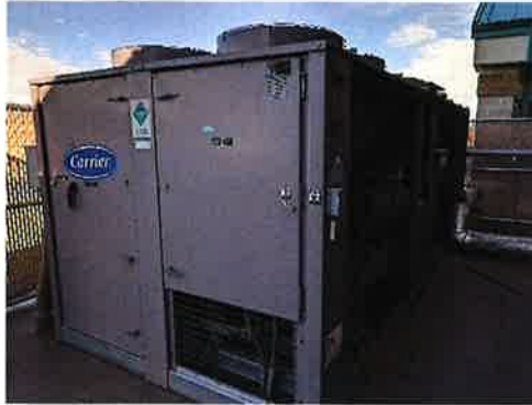
FIGURE 26 – AIR-COOLED CHILLER
