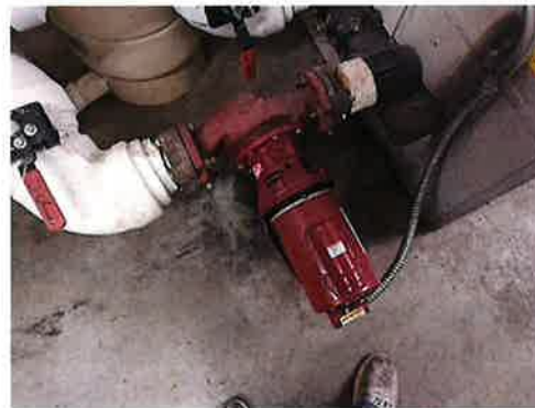
FIGURE 78 – RECIRCULATION PUMP
