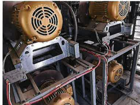
FIGURE 20 – ERU FAN MOTORS
